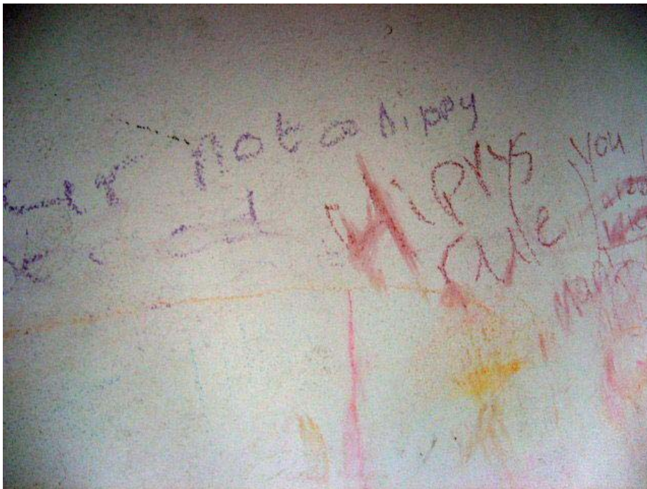
The school wall before
